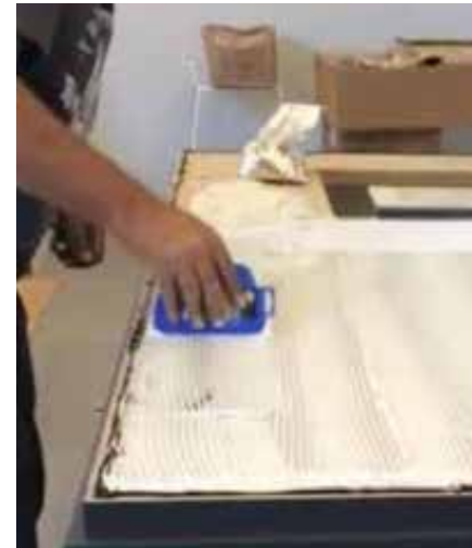
Full coverage of adhesive being applied to substrate
