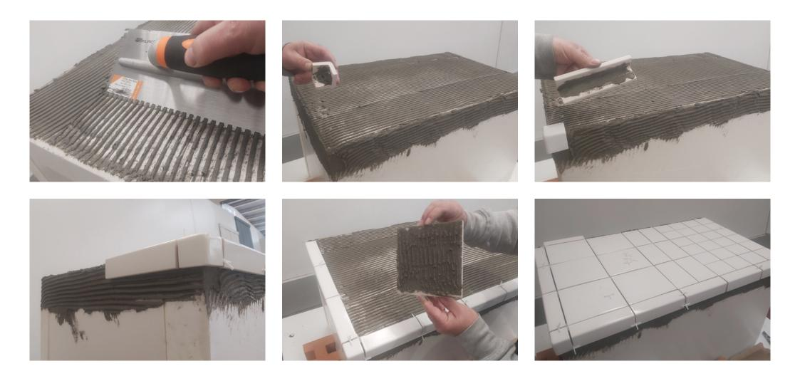
Apply the adhesive with a 5 mm notched trowel, even on corners and edges. Apply the adhesive on all the pieces that are going to be laid. The amount used should allow to adjust the thickness and divide the joints.
