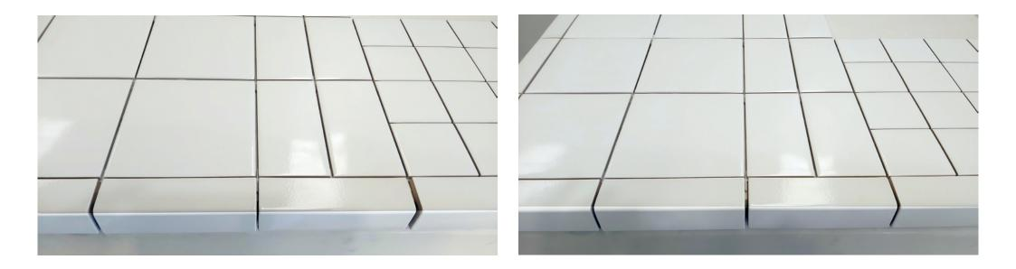
Align the joints properly, dividing them where necessary. Before proceeding with the installation, make sure that the tiling layout has the desired aesthetic effect.
