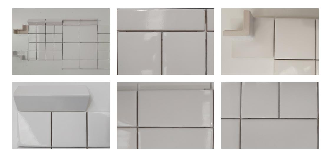
Before installation, verify the dimension of all elements, trying to compensate and divide harmoniously any difference between plain tiles and special pieces.
