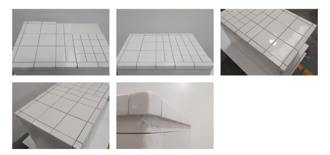
Compose the tiling without using glue. Be sure to consider the thickness of the adhesive.
