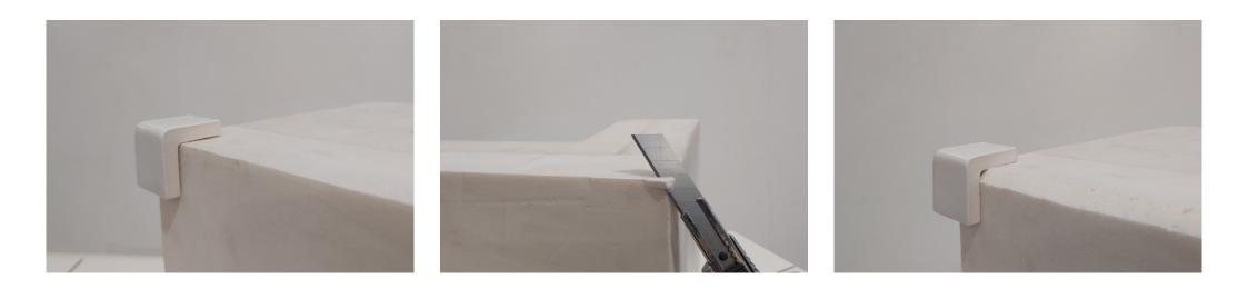
Make sure that all surfaces are perfectly flat. Also, make sure that the corners and edges of any structures are suitably bevelled to adapt to the special pieces.
