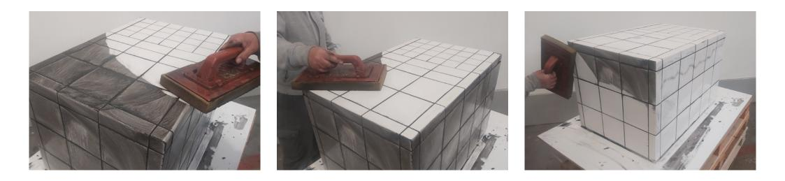
Rinse with water or products suitable for the chosen grout. Make sure to strictly comply with the instructions on the technical data sheet of the product used.
