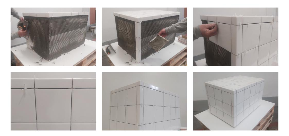
Proceed with the installation, always doing a double layer of adhesive and aligning all joints.
